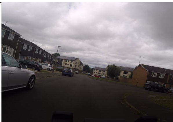
Figure 27 (bottom) – Cornish Crescent - Junction corner radius estimated >9m on internal road
